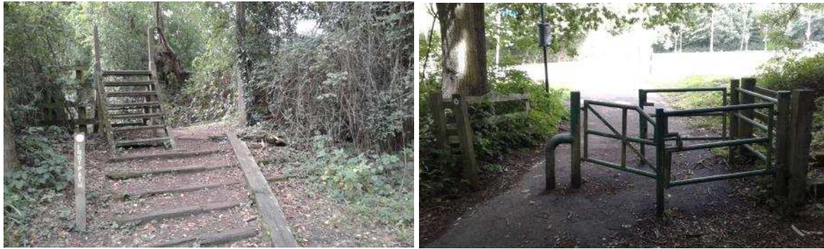
Figure 15. Disused or unnecessary access controls close to Cole Green Station and at Cole Green Lane.
