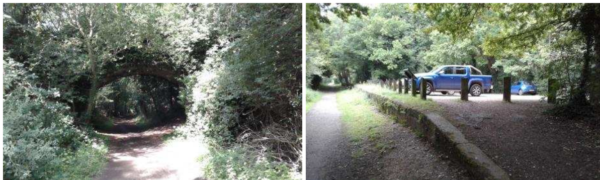
Figure 2. Hertingfordbury Park Bridge and Cole Green Station.
