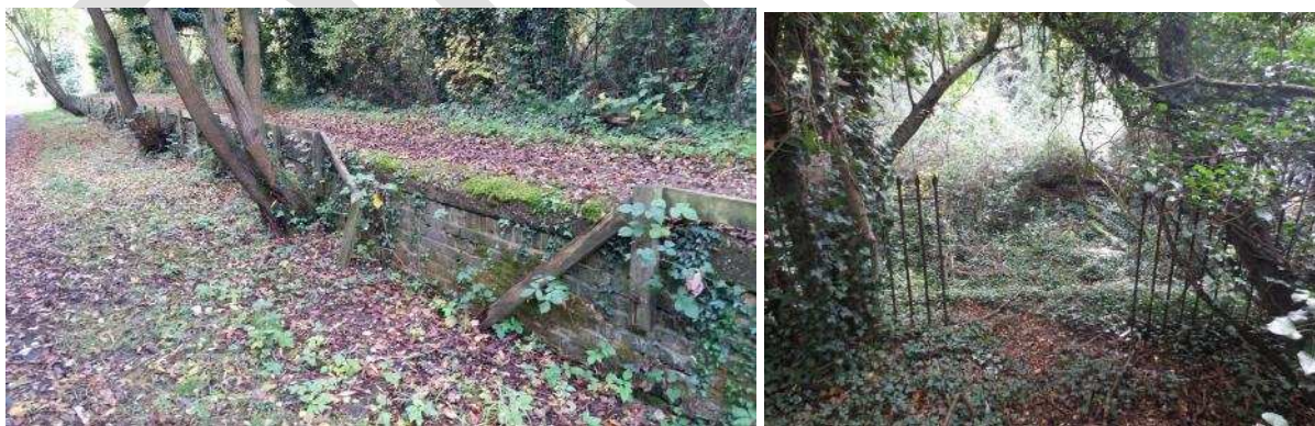
Figure 14. Trees growing from base of northern platform and iron railings within the scrub.
