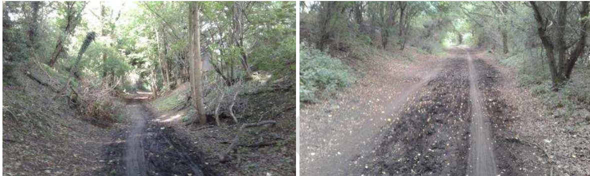
Figure 5. Examples of poor surface, east and west of Hertingfordbury. Sections such as these are often under water during the winter.
